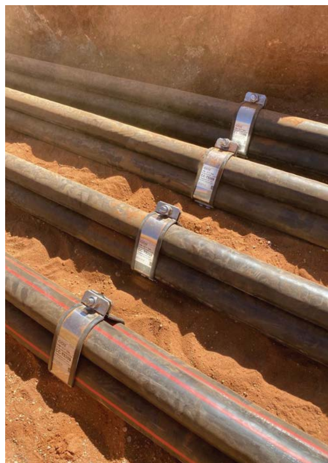
CCG's cleats are designed to withstand mechanical forces caused by fault currents of up to 180 kA.
