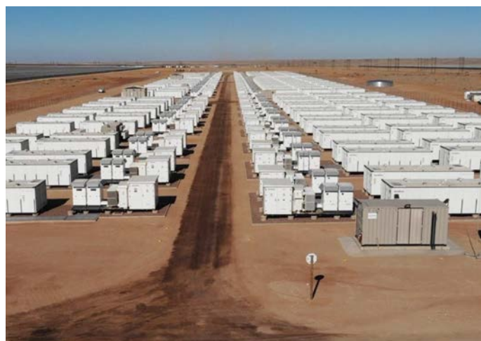
The battery section of Scatec's 540 MW/1 140 MWh Kenhardt hybrid plant.
